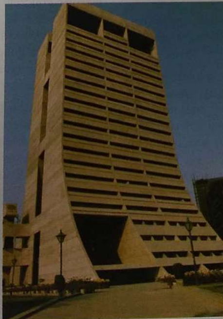
This architecture deliberately displays bare building materials & structural elements and is marked by minimalistic yet voluminous construction
