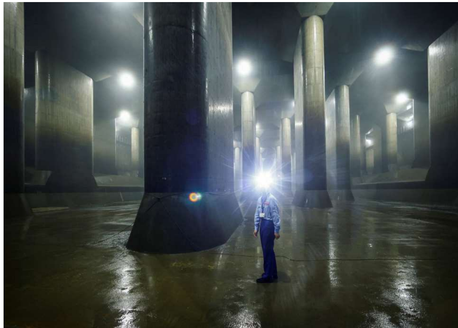
A staff member stands inside a water tank, part of a complex of underground water discharge tunnels built to protect Tokyo and its suburbs against floods during heavy rain, in Kasukabe, Japan. In addition to its engineering ingenuity, the complex is a popular tourist spot and filming location with 59 massive pillars and its own microclimate. The dim interior, punctuated by spears of natural light from apertures in the ceiling, and towering pillars evoke an ancient religious structure. REUTERS
