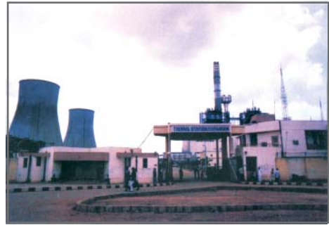
Fig 3.12: A view of a Thermal Power Station
