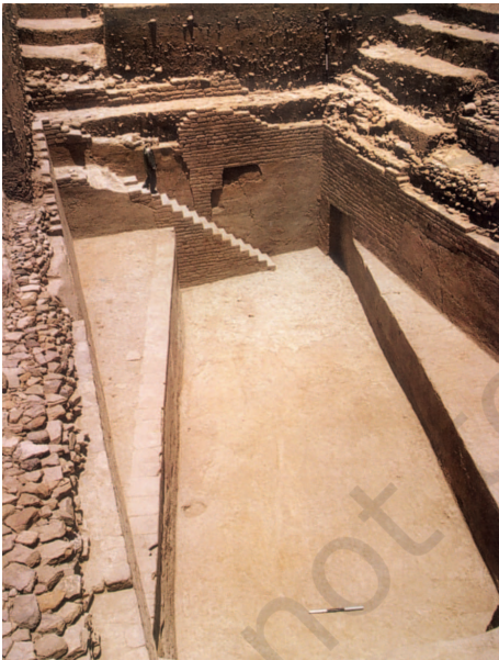
Fig. 1.5 Reservoir at Dholavira Note the masonry work.
