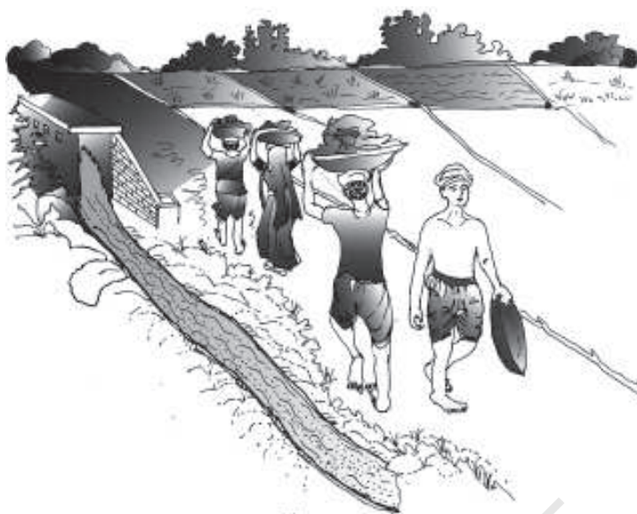
Fig. 7.7 Dam construction work is a direct way of employment generation by the government
