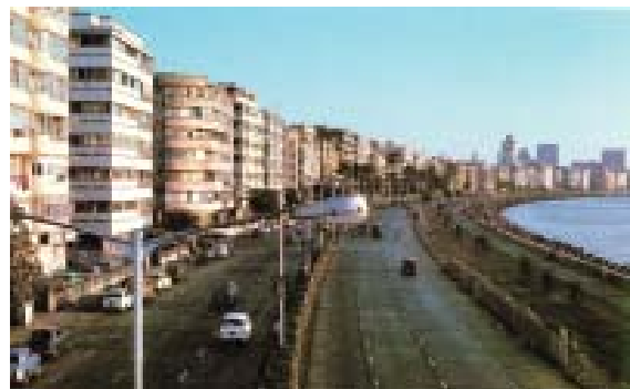
Fig. 23 – Marine Drive. A familiar landmark of Bombay, it was built on land reclaimed from the sea in the twentieth century.
