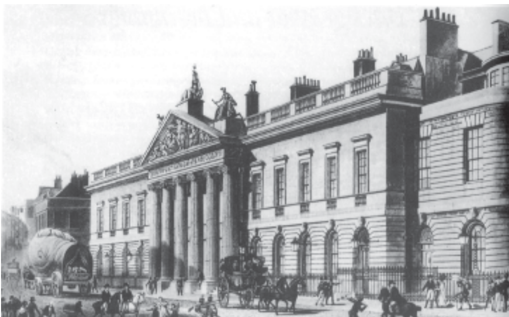
Fig. 17 – East India Company House, London.
