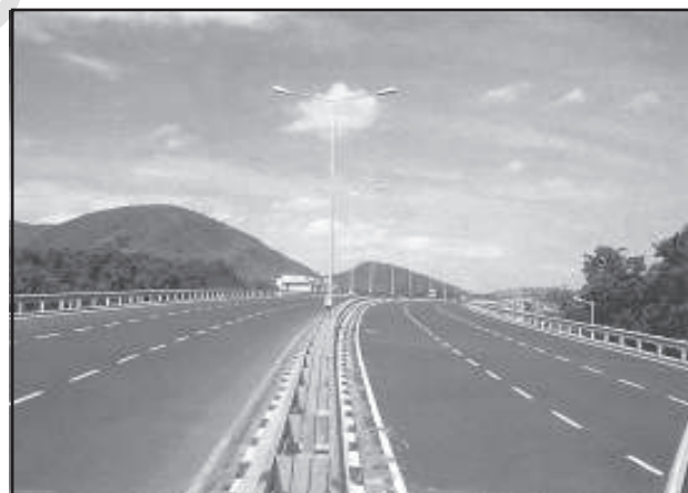
Fig. 8.3 : Dharmavaram Tuni National Highway, India
